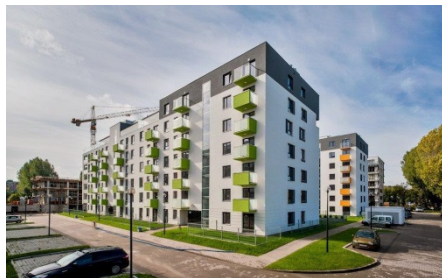
Osiedle-Innova (stage IV). Date of delivery: September 2013. No. of units: 92 apartments (4,468 sq. m).
