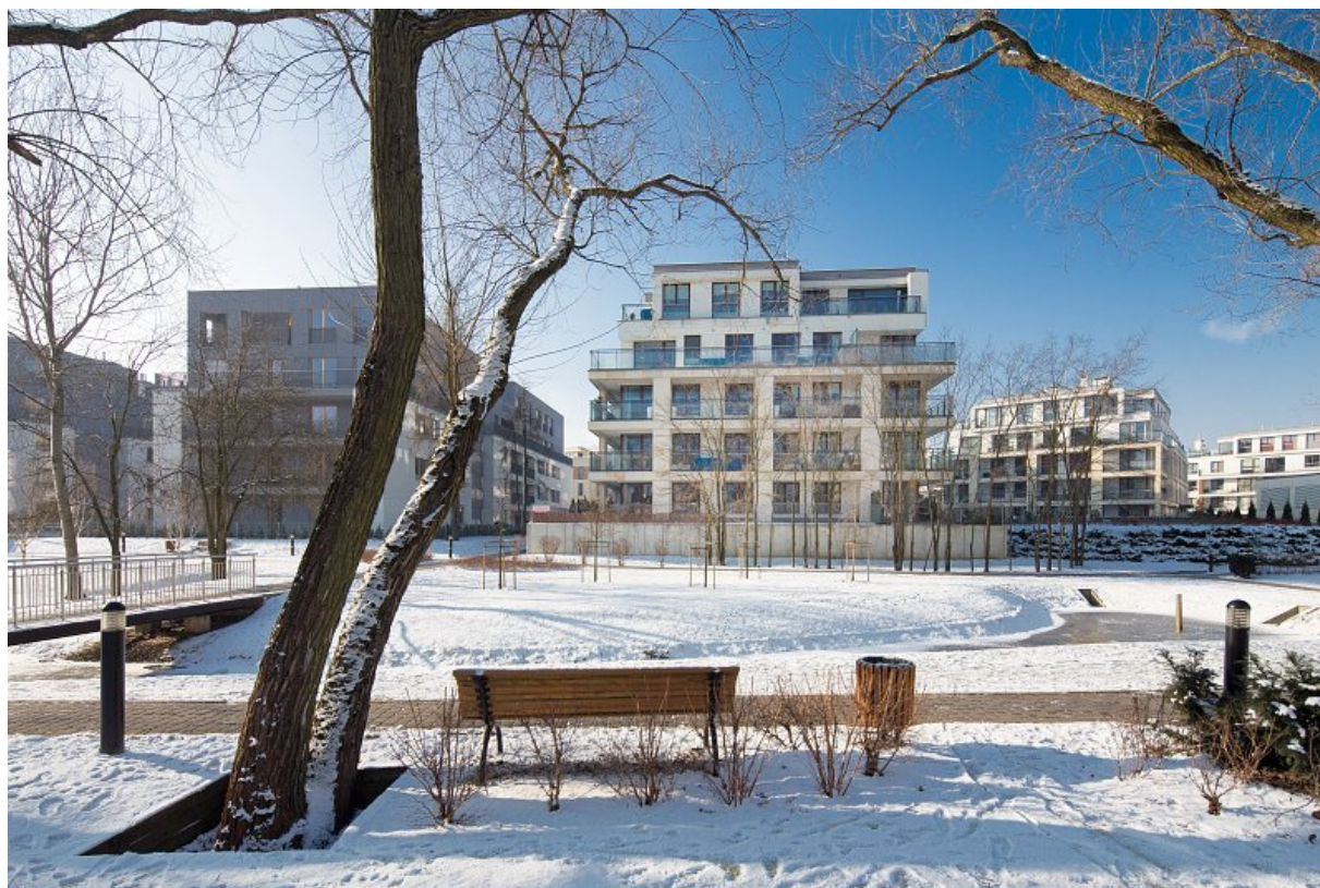
Buildings C2 & C4 by the central lake in Ostoja-Wilanów real estate (Warsaw) (February 2018).
