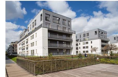
Ostoja-Wilanów (stage 6.A, building C2). Date of delivery: November 2016. No. of units: 120 apartments (12,531 sq. m). Presold: 99% (as at 30 September 2017)
