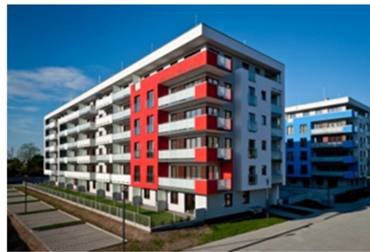
Osiedle-Innova (stage II). Date of delivery: June 2012. No. of units: 71 apartments (3,757 sq. m).
